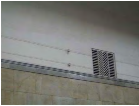
Shows 'leaky feeder' in close up
